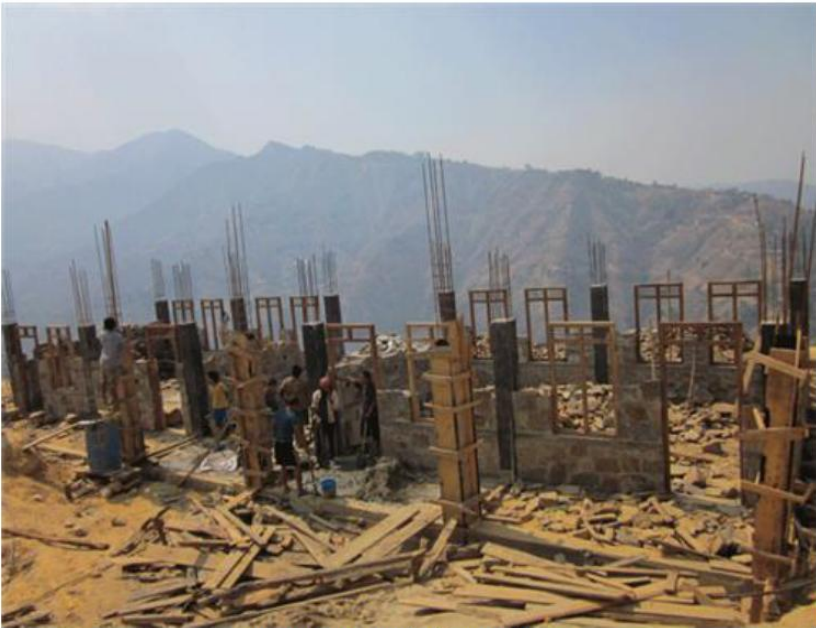
Construction work of ground floor.
